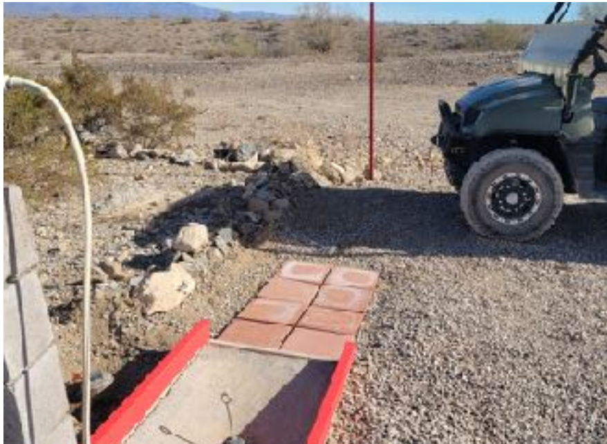
RV dump station upgrade
